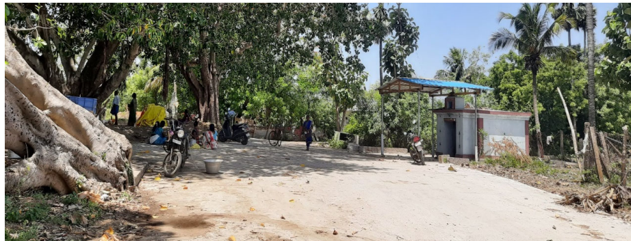
Lack of street light at junction point @ Illanthoppu
