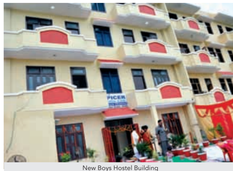
New Boys Hostel Building
